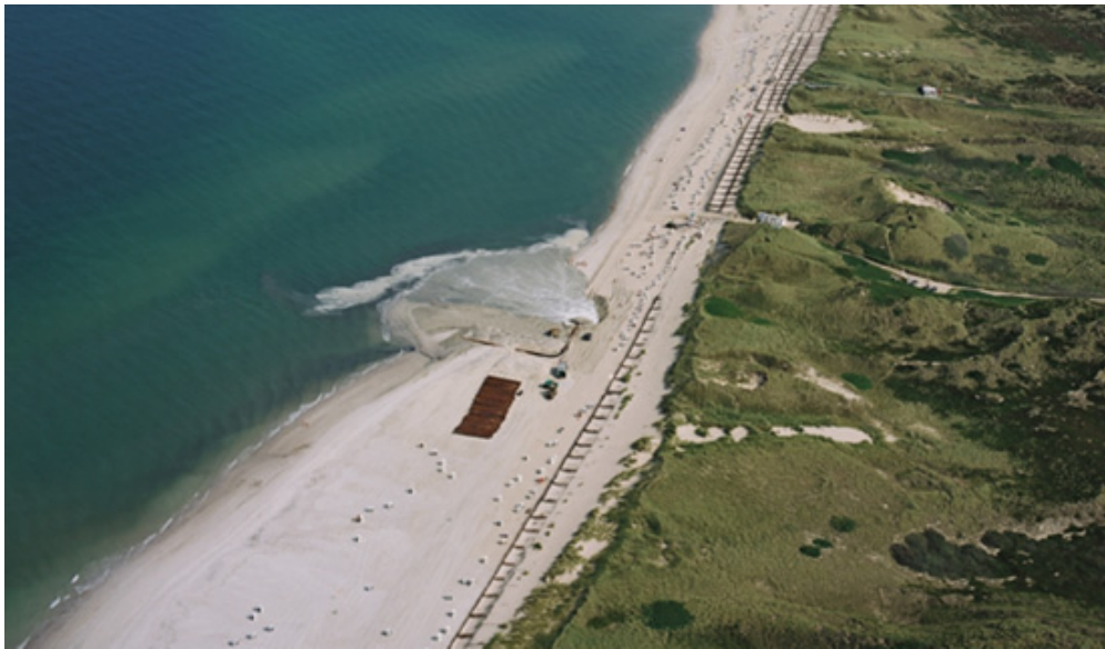
Figure 5: Sand nourishment on the island of Sylt (Germany)
